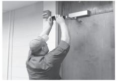
**STEP 2:** Slide the device over the door closer to secure the door.
